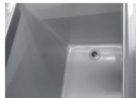
5. From the outside secure the drain with the washer and nut.
