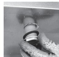
6. Tighten the nut with channel locks, use a fork to hold the drain in place if necessary.
