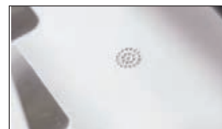
Each compartment has a floor drain for quick drying after cleaning.
