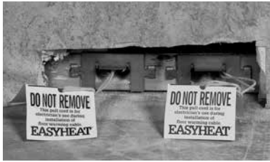
Figure R6. Fish cord installation
