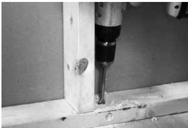
Figure N4. Fish hole preparation
