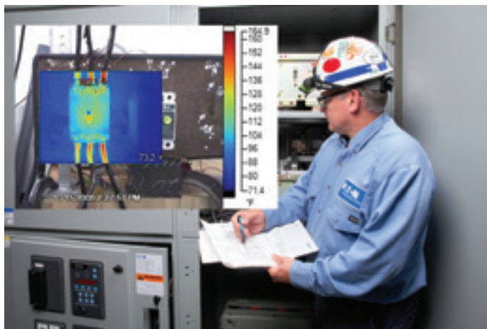
Figure 4. IR cameras can be used to provide insight to see breaker health.
