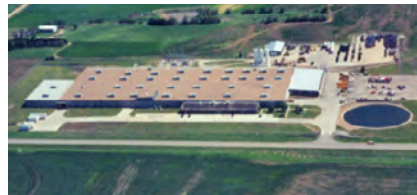
Hoisington Communications Plant | Hoisington, KS
