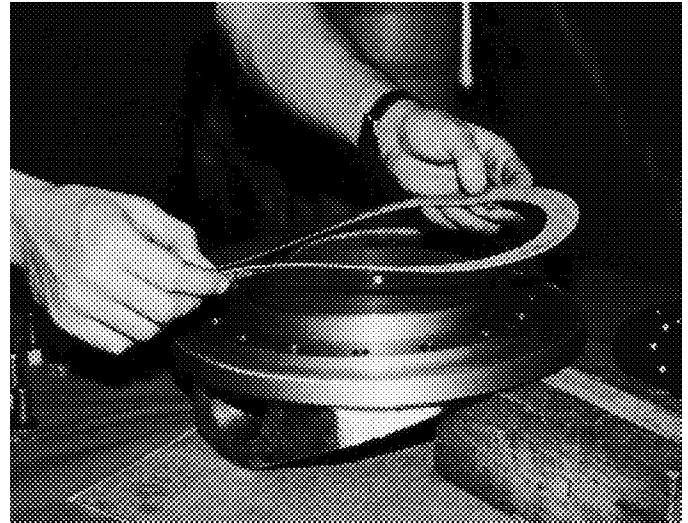
Installing the Gasket
